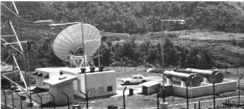
**Figure 1.5** Palapa A light-traffic earth station (10-m antenna) in Indonesia.
