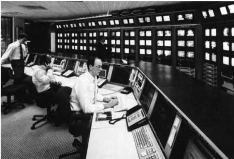
**Figure 11.2** Network operations group of a satellite operator, the control point for access to satellite transponder capacity; it may also serve as the management point for part of the ground segment.
