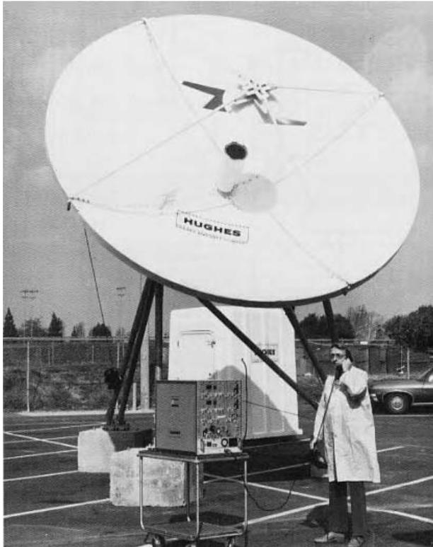
**Figure 1.6** A 4.5-m earth station capable of telephone service (circa 1977).
